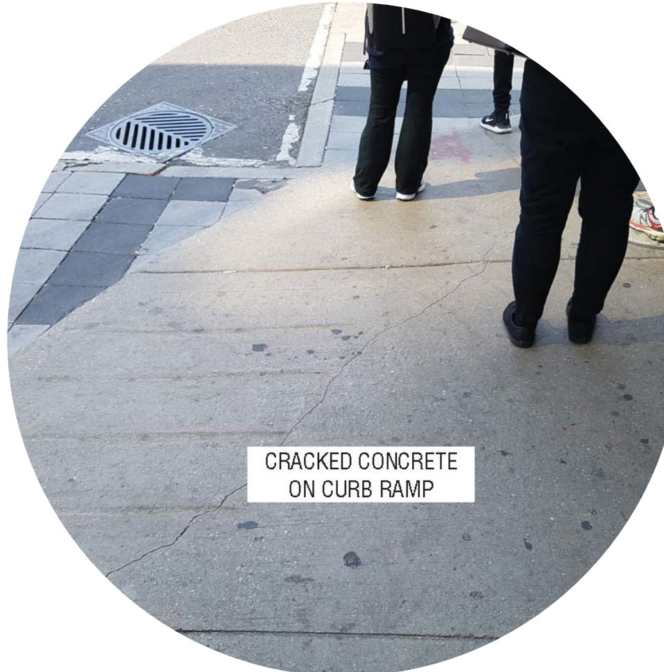
No tactile warnings at curb ramps
